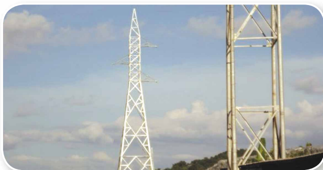
A Captive Power Generation Plant financed by the Bank through Ganeshguri Branch under Guwahati Regional Office
